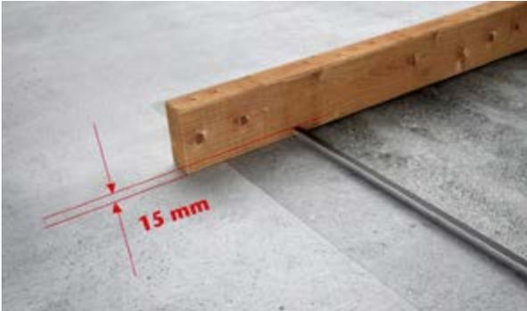
**Step 7:** For recessed covers ensure reinforcement provided is correctly positioned. Haunch the frame fully with concrete (minimum 150mm wide) and fully fill the cover to within 15mm of its upper surface. Use a notched batten to help level concrete. Vibrate concrete where necessary to ensure no voids. Minimum grade C35/45 concrete to BS EN 206:2013 (maximum aggregate size 10mm). Recommended slump S2 or S3.
