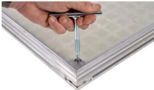
**Step 2:** Unscrew and remove the locking screws with the lifting/locking keys provided. Take care when unscrewing the locking screws on ASSIST versions as the cover may start to open automatically once the screws are unfastened. If this happens simply hold the cover in place until ready to be fully opened.
